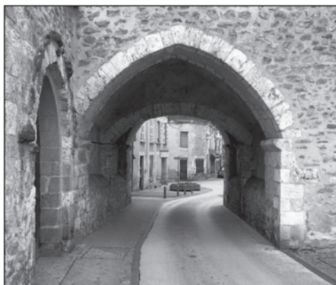
Le Belfroy construit au XIII e siècle The Belfry built in the XIII th century
